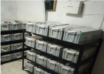
10 Kva Inverter Installation at a Bank branch in Calabar, Cross-River State
