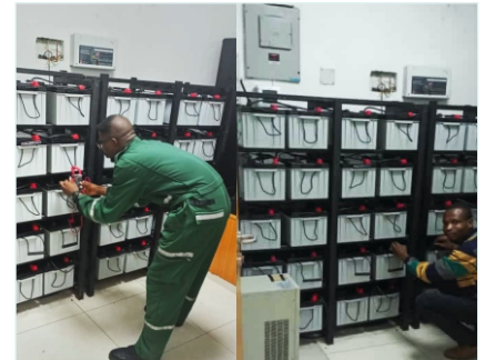
10kva Inverter Installation for a bank branch in Asaba, Delta State, Nigeria
