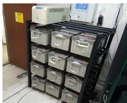
6kva Inverter Installation at a Bank Branch in Port-Harcourt, Rivers State
