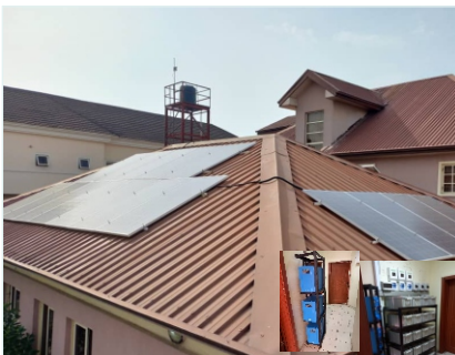
10KW Residential Solar Installation at Lekki, Lagos
